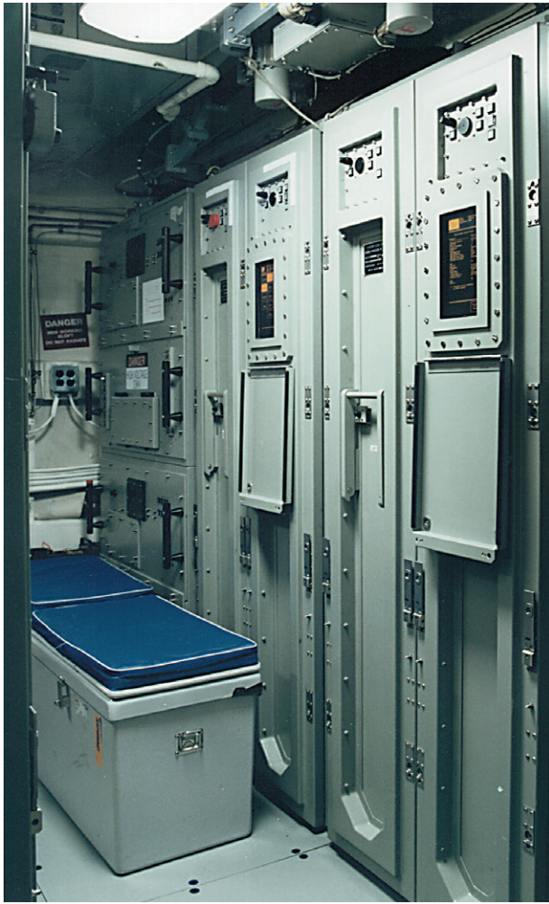
Figure 4. CEC equipment installed on the USS Cape St. George . Shown are the cabinets that house the CEC electronics.
