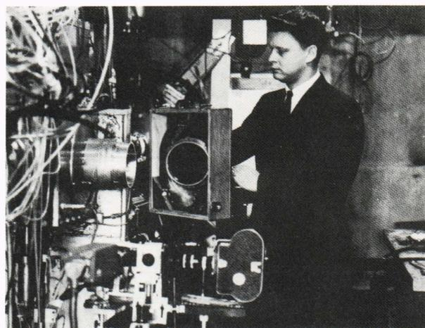
**Figure 7.** Frederick Billig stands beside the Mach 5 wind tunnel in which he conducted the first successful test of an external-burning ramjet model.
