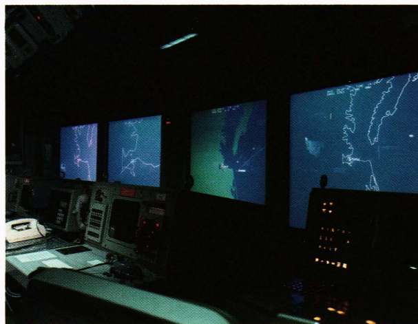
Figure 1—The large-screen color display for the Command Support at-Sea Experiment, installed in USS Yorktown .
