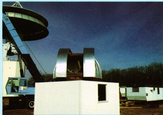
The APL Solar Observatory near the 60-foot satellite tracking antenna. The building houses a Zeiss telescope with a photoelectric guider. The telescope is mounted on a cement pier set 10 feet into the ground in order to limit vibrations. A PDP 11/23 computer has been installed at the observatory for data recording and instrument control.
