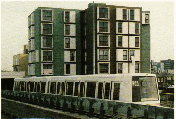
Automatic guideway transit application in France, connecting Lille to the new town of Villeneuve d'Ascq. (Photo courtesy of P. Smith.)
