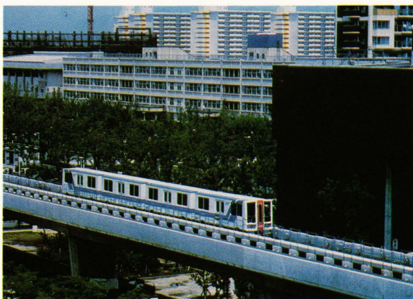
Automatic guideway transit application in Osaka, Japan, connects a man-made island in Osaka harbor with the mainland. In the background are residential units on the island. (Photo courtesy of K. Morita.)
