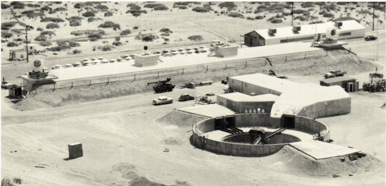
The Talos Land System, installed at White Sands Missile Range, included two C-band monopulse radars, two C-band guidance radars, a launching system, and a partial magazine for six missiles.
