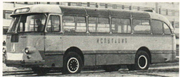
Fig. 5—Soviet flywheel/engine hybrid bus (circa 1971).
