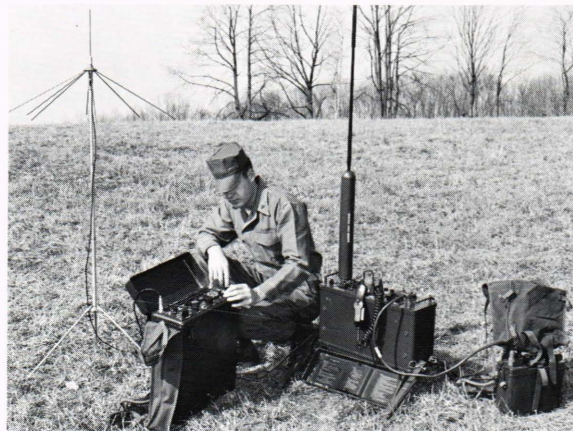
Fig. 5—Experimental translocation receiver (left) and auxiliary communications transmitter (right) at forward observer station.
