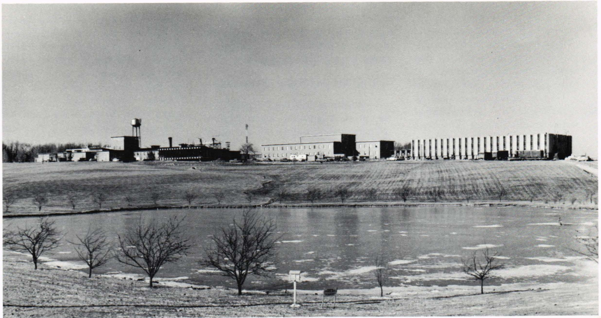
Main building complex of the Howard County site of the Applied Physics Laboratory. The new Building 4 (right) and Library (center) are shown in late stages of construction.
